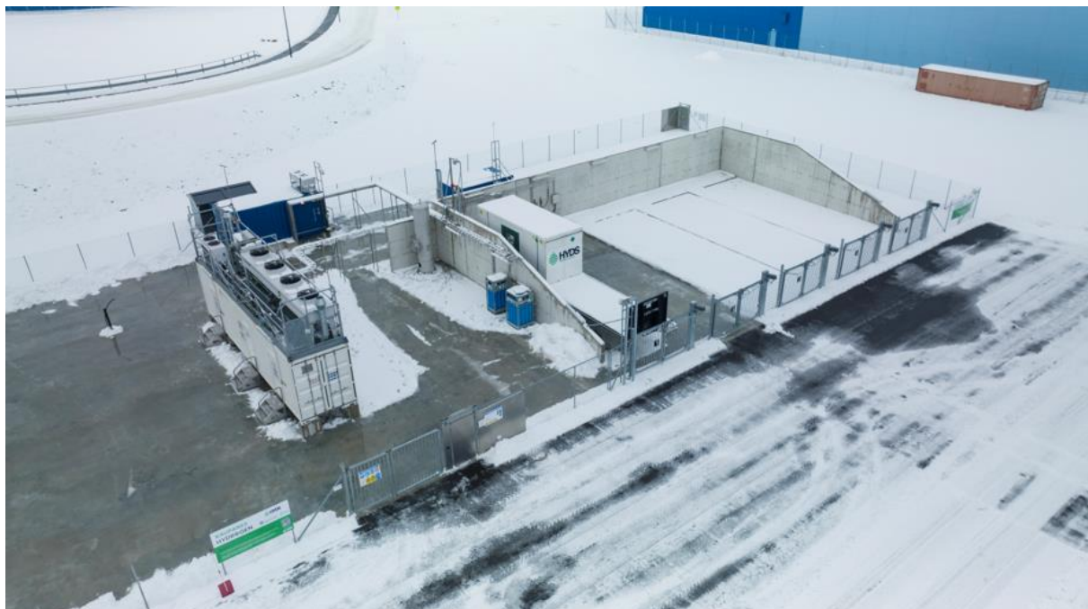
Figur 4-1 Kaupanes hydrogenanlegg. Kjelde: HYDS
